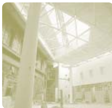
The Experimedia courtyard in construction
