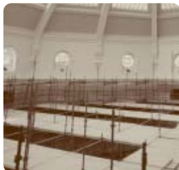
An interior view of the Dome shortly after the installation of the skylights
