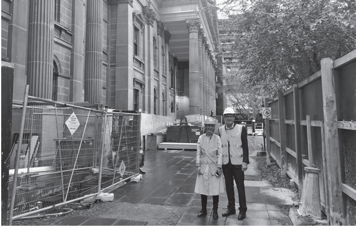
State Library CEO Kate Torney and Board President John Wylie at the Swanston Street entrance construction site.
